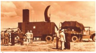
WWII, the GCA Fig. 1 The AN/MPN-1, the world's first GCA, was Gilfillan's entry became famous into radar.
